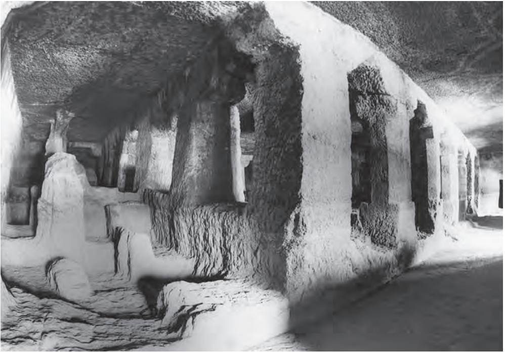
(159) Ajanta Cave 24 interior. View from front left corner, 475-477. The unfinished interior of the huge Cave 24—abandoned at the end of 477 when the great emperor died—is a virtual laboratory for the study of excavation techniques. The cutting of course progressed, in general, from the top down and from the front to the back; all work must have been done by contract, with payment being made when certain given areas or forms were done.
