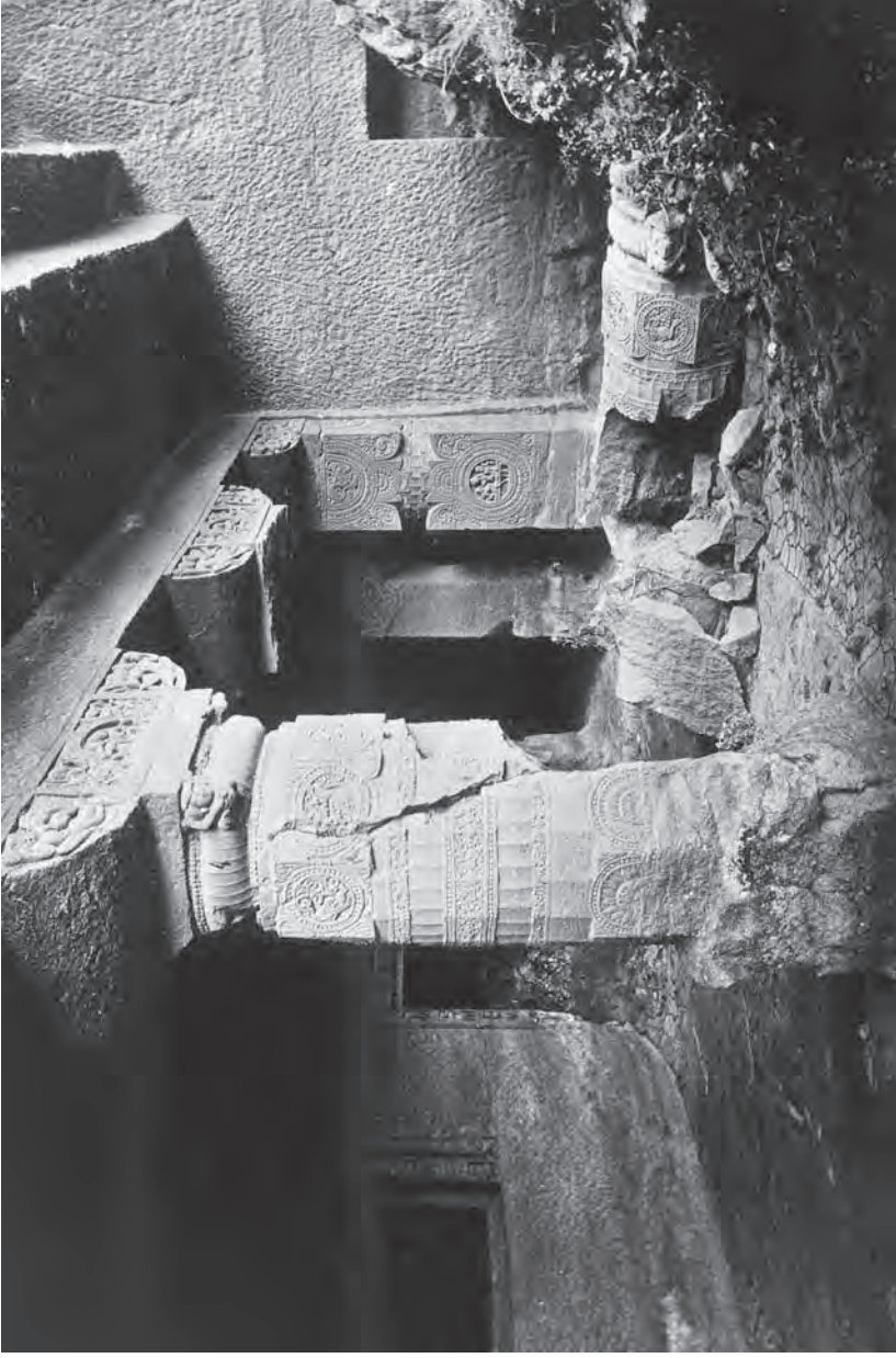
(152) Ajanta Cave 24 porch. Broken colonnade, 475-477. This photograph, taken over a century ago, shows the state of the beautiful Cave 24 as it appeared in early days. The damage was caused by the pervasive flaws, which caused so many problems for the excavators. Here, we can see a particularly bad one running between the lava layers more or less horizontally, just below the splendidly carved capitals. Over the centuries deep debris—here some five feet—built up in porches such as this, and as it dried (and contracted) and then became wet (and expanded) from season to season, it gradually displaced (millimeter by millimeter) the flawed shafts, until they literally toppled over, generally leaving the capitals above intact. Unhappily, many years ago, in some misunderstood effort at a “clean-up” of the site, all of these splendid fallen pieces were thrown into the nearby river.
